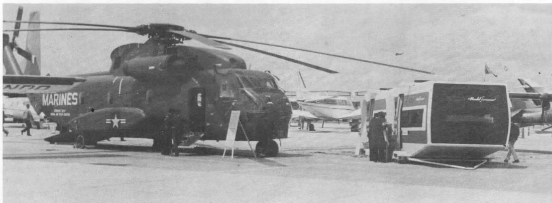
U.S. Marine Corps/Sikorsky CH-53A on static display at the 27th Paris Air Show this month. To the right of the aircraft is static display of the Budd Company's Skylounge prototype, the XB-1. The experimental module is the forerunner of a 40-passenger pod, which would be transported by an S-64 Skycrane. The Skylounge study is currently underway for the city of Los Angeles.
